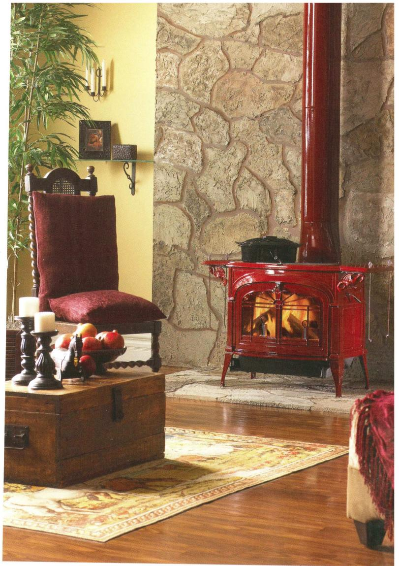
**ABOVE:** A masonry heat shield and insulated hearth like this faux stone arrangement is a deterrent for fire and also protects the wall framing and floor from intense heat.
